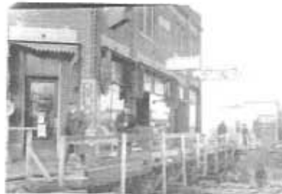
Moving operation for wider Woodward , 1924. The Aston-Wallace Building (which still stands today at the corner of Troy and Woodward) was moved west and south from Nine Mile Road. ----- Ferndale Historical Museum Collection
