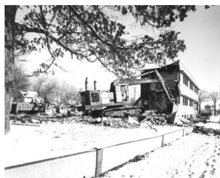
Demolition of Ardmore Hospital, 1989
