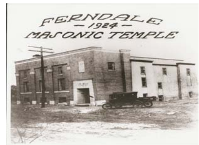
Ferndale's Masonic Temple Nine Mile/Planavon 1924
